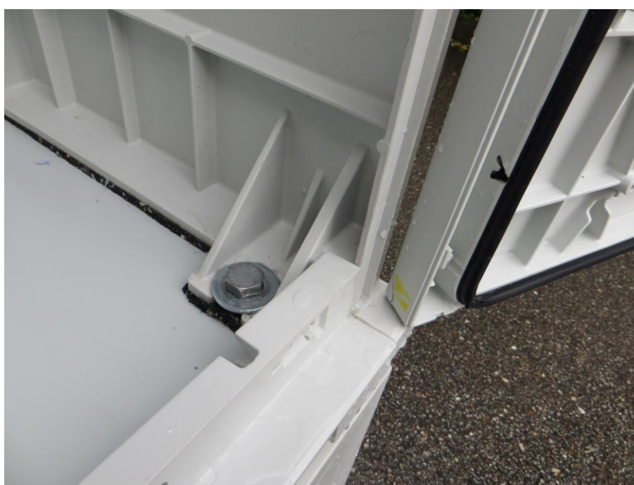
unsignificant penetration of water around the door
